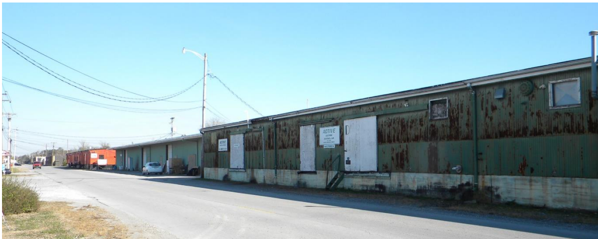
Industrial buildings along interior streets
