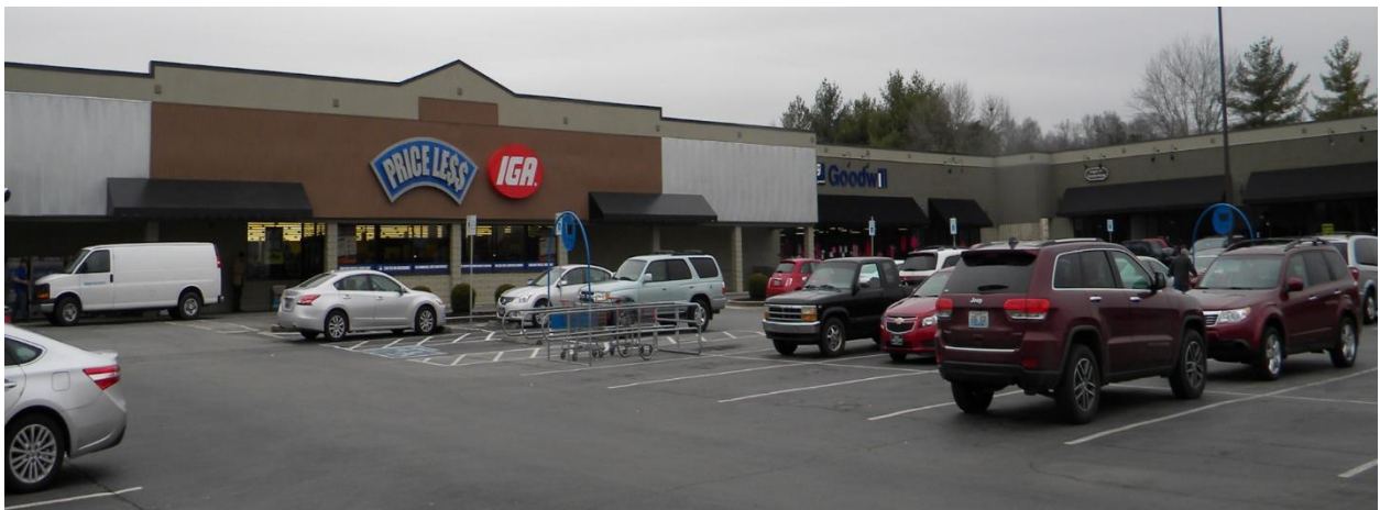
The neighborhood shopping center on Emory Valley Road at Briarcliff Avenue.
