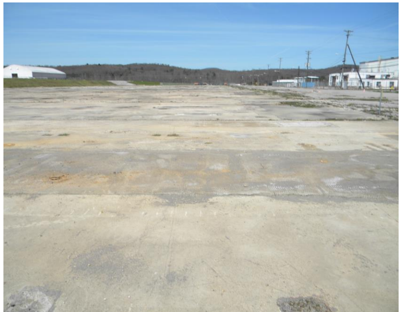
Part of the K-25 slab
